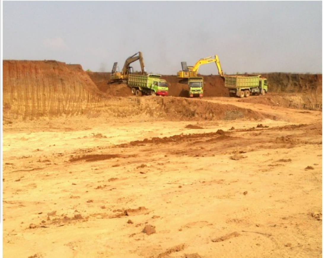
Cut and Fill Work in Phase 3
